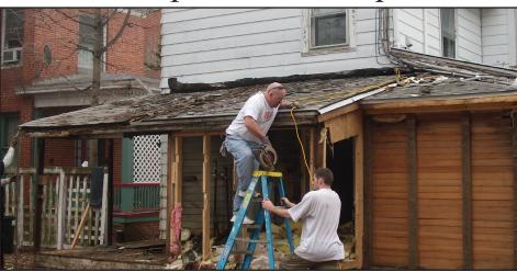
Mid Shore Exteriors is schedule to replace the building's roof during the week of February 22, 2011. The entire roof will be removed and new plywood and roofing shingles will be installed and will take approximately two days to complete.
