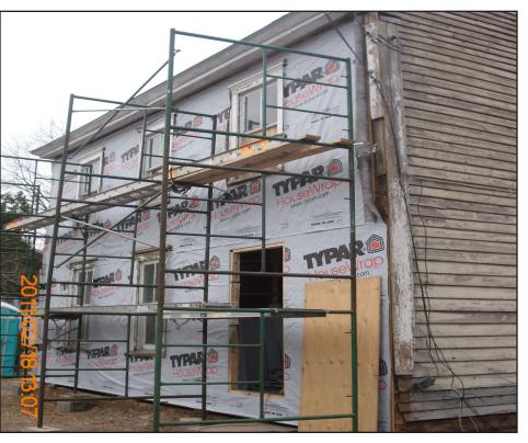
Exterior renovations are in their third week. The building is nearly stabilized with the replacement of all of the building sill plates.
